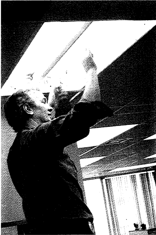
1a. The fluorescent tubes on both sides of the heat shield are removed for access to the ballasts.
